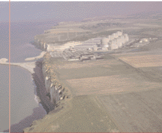
Paluel unit for nuclear electricity production.
