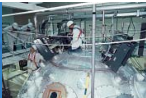
Work on the laser integration line's experiment chamber, prototype of the future Laser Megajoule, Le Barp (Gironde).
