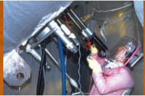
Servicing work on power plant steam generator tubes.
