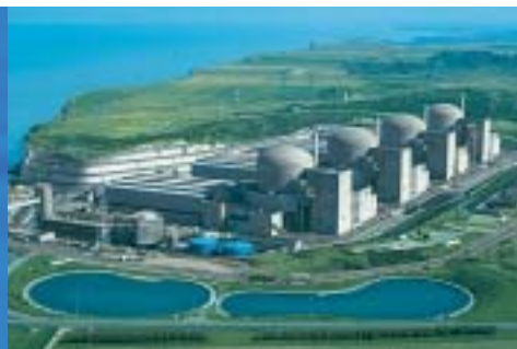
Paluel nuclear electricity power plant (Seine-Maritime).
