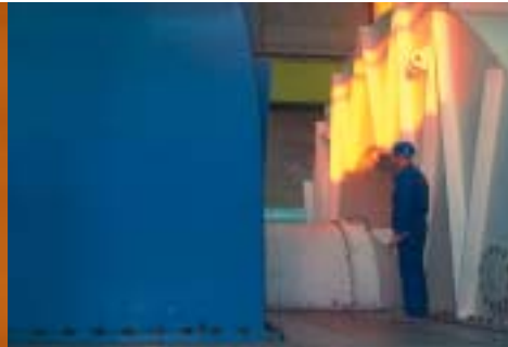
Turbogenerator set, overhaul at the Le Blayais power plant (Gironde).
