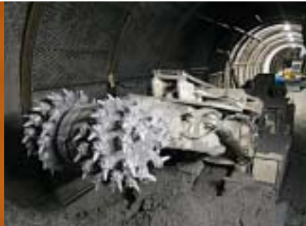
Head of the roadheader excavating machine.
