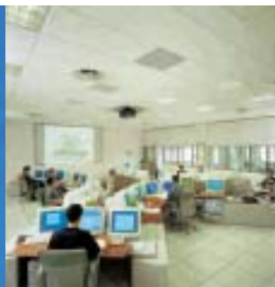
The installation's control room.
